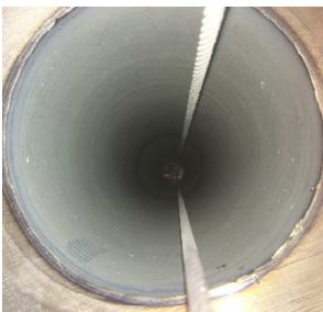
Ripple internal welding
